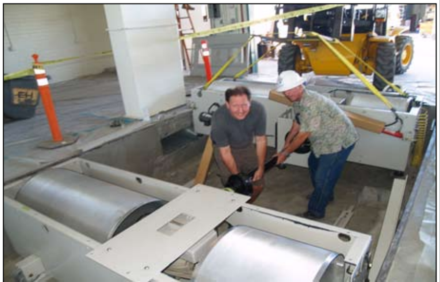
Auto Shop at Nogales: Automotive teacher Mike McCarthy and Erickson-Hall Construction Superintendent Bob Lathrop Sr. install a new chassis dynamometer for testing overall car operation. The facility opens this Fall and offers students interested in a technical education in the auto industry the opportunity for state-of-the-art learning experiences.
